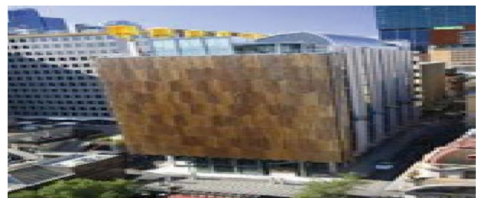
Figure 5: Council House 2 building in Melbourne 17 .
